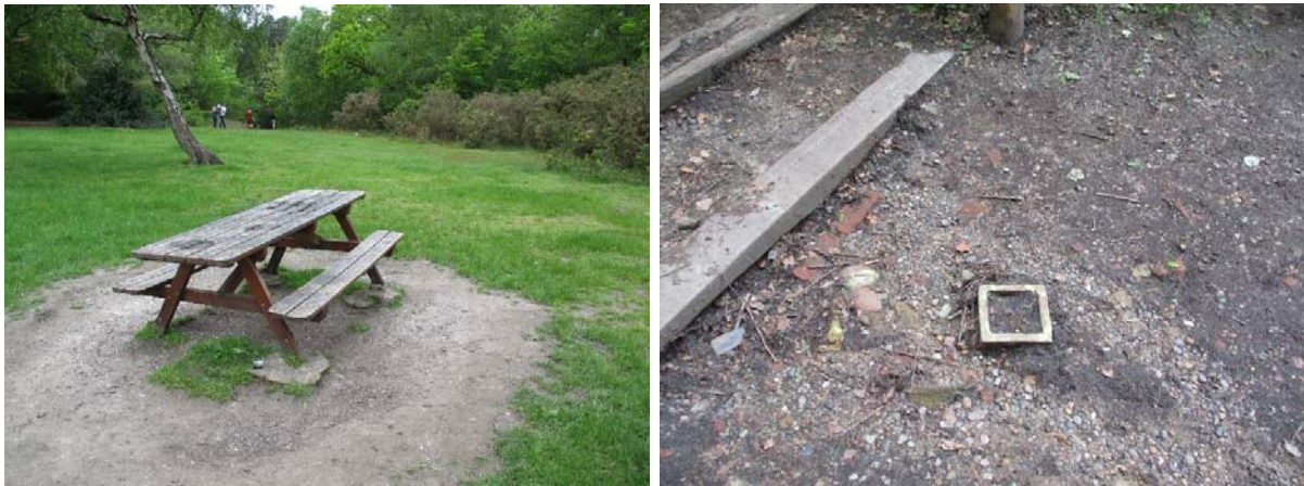
Figure 11. Furniture or features used by or accessible to the public that may need repair or removal/replacement, including fire-damage bench and exposed hydrant cover near steps.
