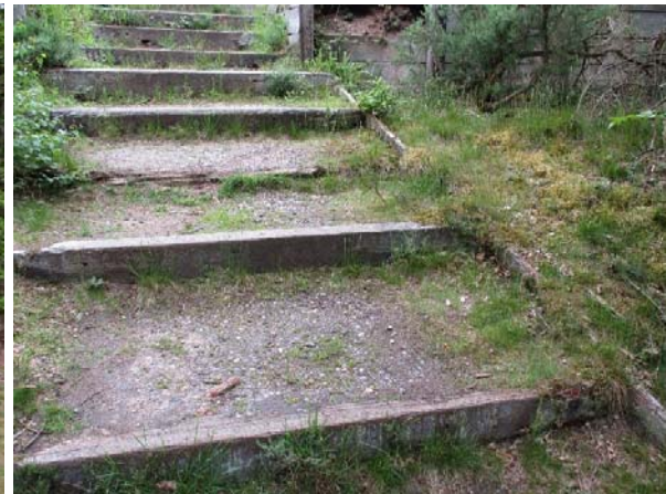
Figure 5. Degrading wooden steps on part of Keston Common, which pose a growing accessibility issue for less abled users.
