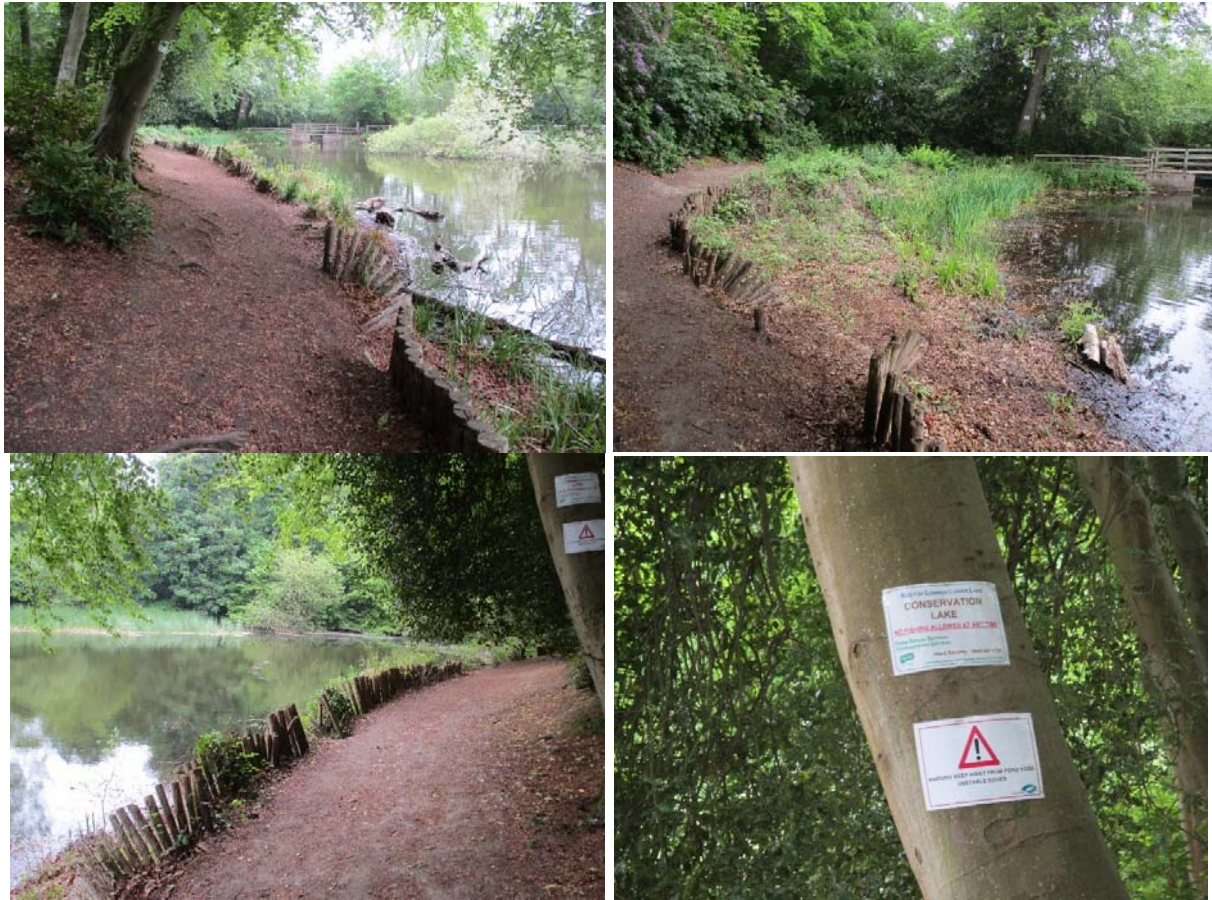
Figure 8. Sections of path alongside the western side of the upper pond, which is suffering from continual erosion and progressive bank collapse into the pond.
